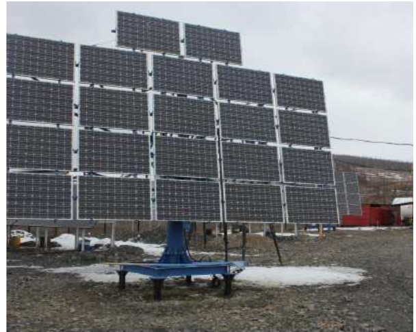
10 kW automatic solar tracker in Yuchugei, Oimyakon ulus
