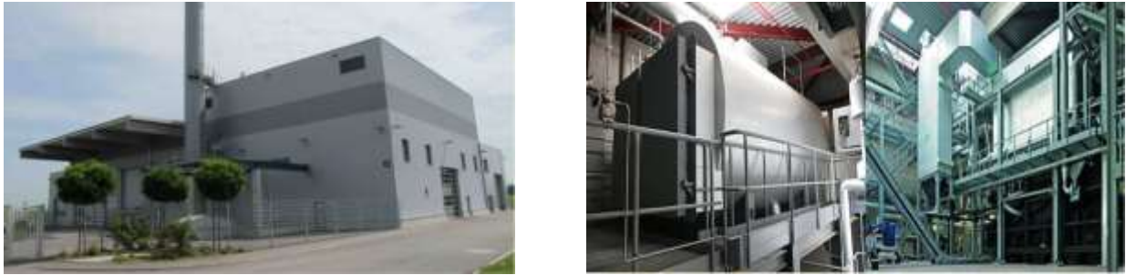
Figure 4.23 Exterior of boiler-house with organic Rankine cycle turbine
